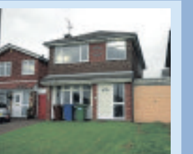
7 DUGDALE CLOSE, CANNOCK
